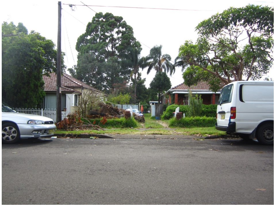
Figure 12 – 66A Beauchamp Street viewed from the street
