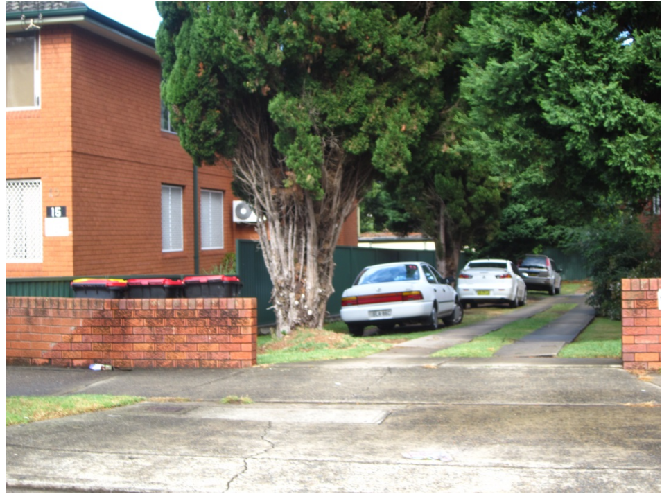
Figure 2 – 13A Denman Avenue as viewed from the street
