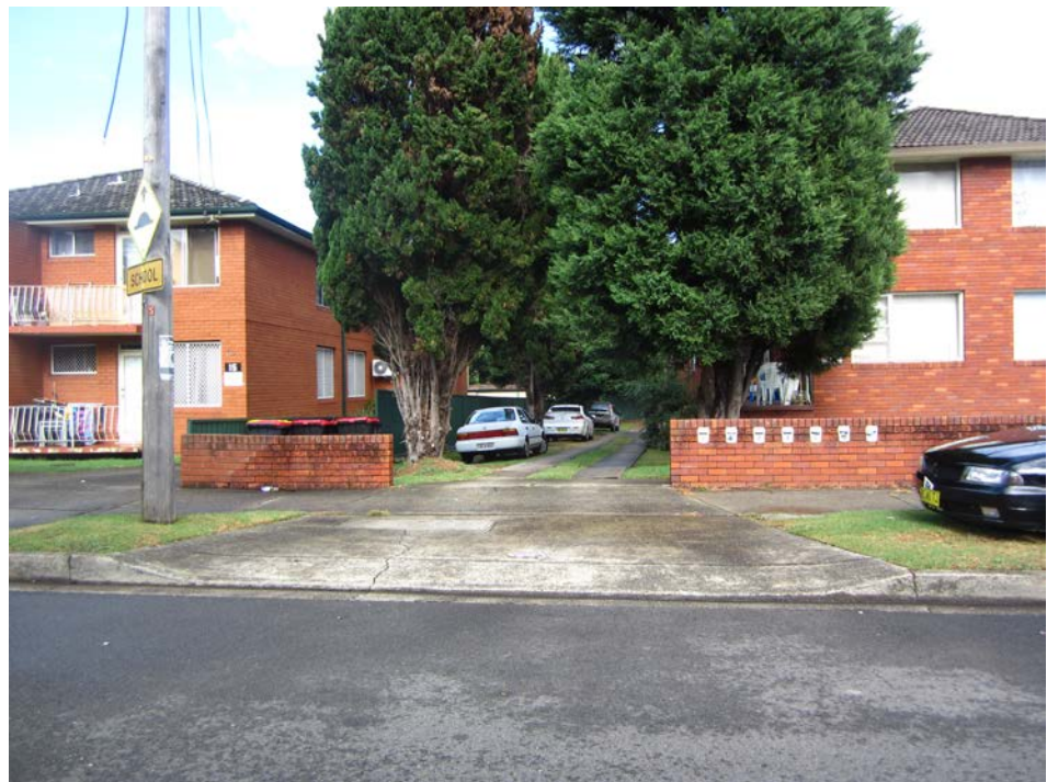
Figure 3 – 13A Denman Avenue in context
